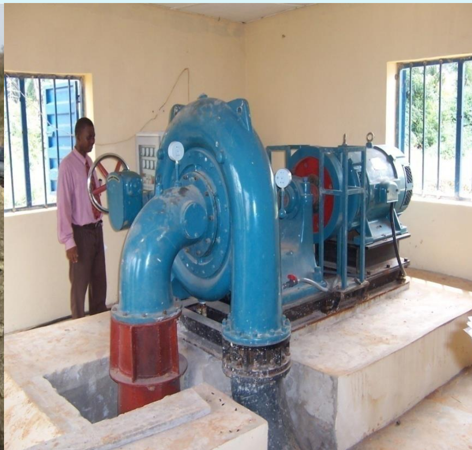
Penstock bifurcation into the 2x75 kW Francis Turbines house at Waya Dam, Bauchi State installed by UNIDO
